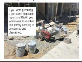
that high winds during storm events don't knock them over. Make sure that they are fitted with a containment tray and that it has ample capacity to capture a spill.
